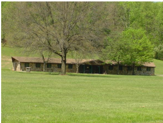
Outside View of Cottage
