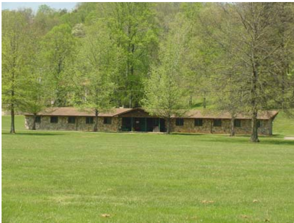
Outside View of Cottage
